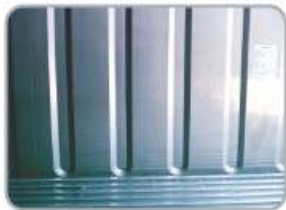
Inside Wall : Corrugation
